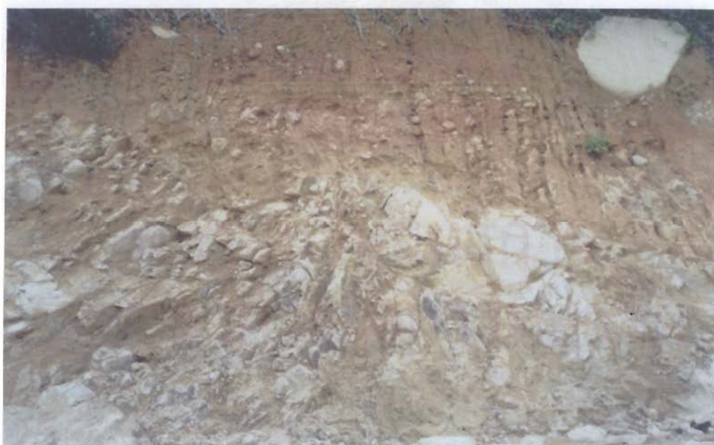
Figure 4.3b Residual soils and weathered granitic rock along Highway number 4233, Grid Ref. 196E 781N.
