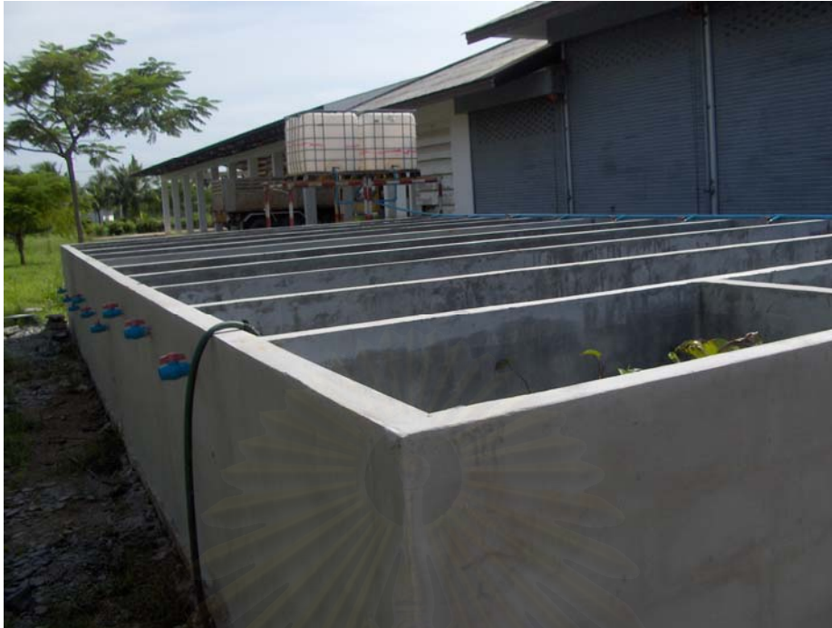
The Constructed Wetland
