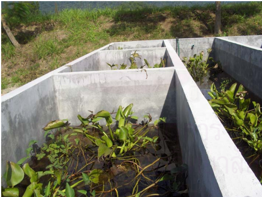
Stabilization of New Ponds with Normal Water, Water Hyacinth, and Morning Glory
