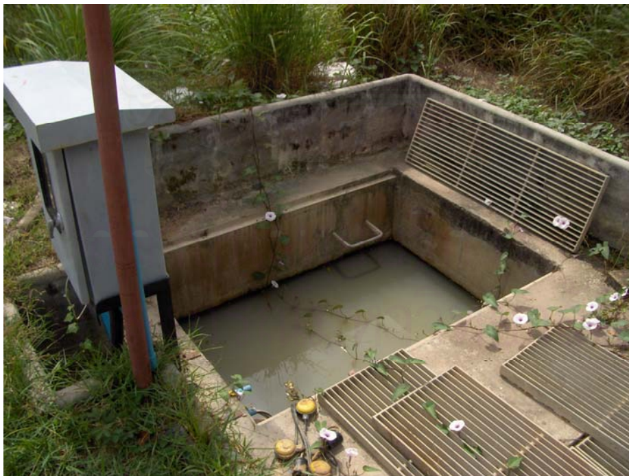
Manhole of Saensuk Municipal Solid Waste Disposal Center
