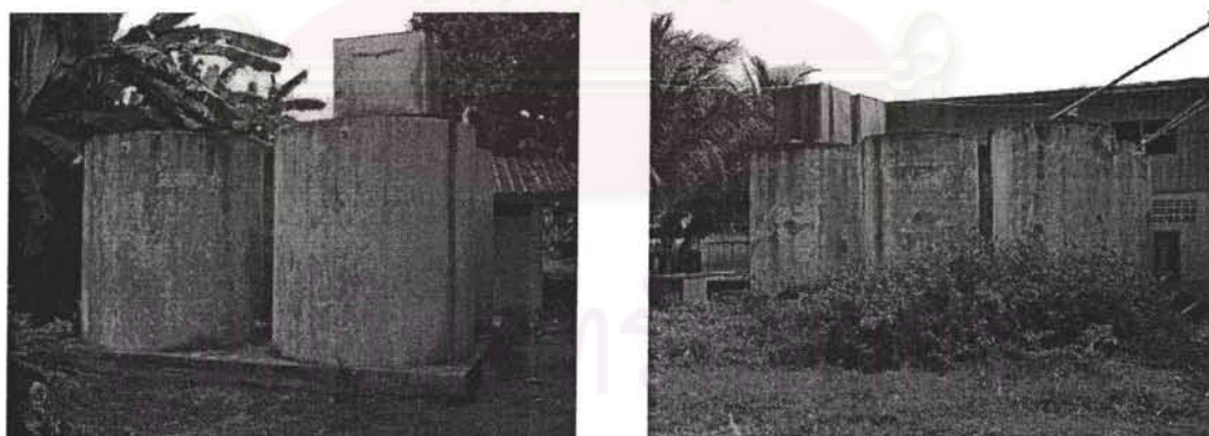
Figure 6: Previous Water System for Drinking Water at School
