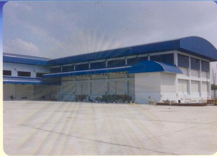
COLD STORE ROOM
