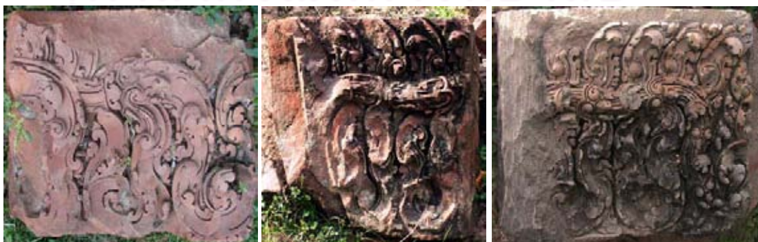
Figure 2- 8: Fragments of Lintel spreading inside the enclosure wall. (photo in 2009)
