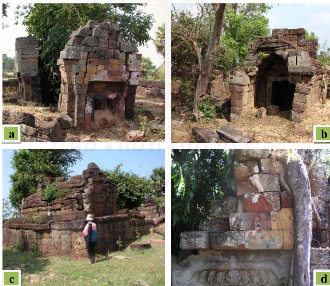
Figure 2- 10: (a) Main central sanctuary; (b) laterite edifice of library; (c) Laterite enclosure wall and (d) Fronton at the west of main sanctuary. (Photo in 2009)
