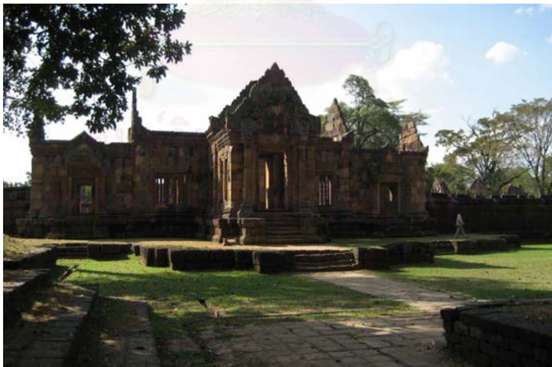
Figure 3- 13: Eastern main gopura of Prasat Muang Tam. (photo in 2009)
