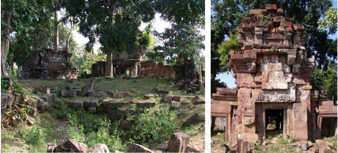
Figure 2-2: Viewing from the disappeared central sanctuary to library edifices at the East (left) and the Eastern gopura (right). (photo in 2009)
