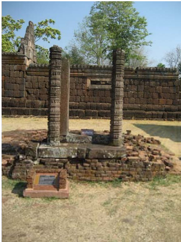
Figure 3- 3: Ruined brick building, northeast of main sanctuary. (photo in 2009)
