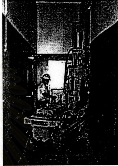
Micropiles earthquake proof Robinson May Department store in Northridge at Laurel Plaza.
