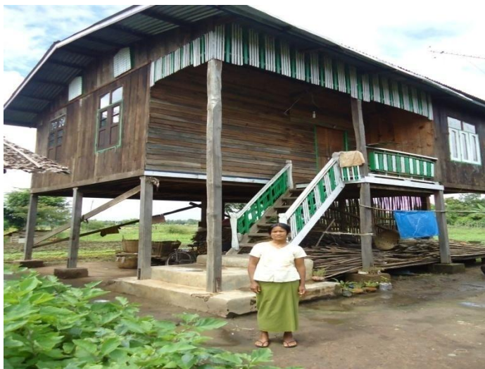
1.7 Daw Aye Cho Sat with her renovating house.
