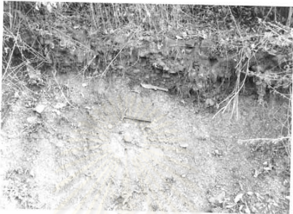
Fig.3.5. Residual weathered basalts overlies gravel deposit of the Triassic rocks at the west edge of the Sop Prab-Ko Kha basaltic area (grid reference 357914).
