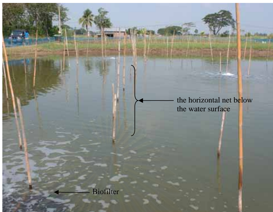
Figure 3-10: The treatment pond containing biofilter sets and horizontal net
