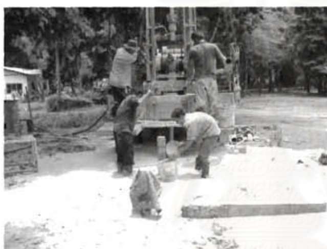
Figure 6.3 Borehole drilling for samples collection.
