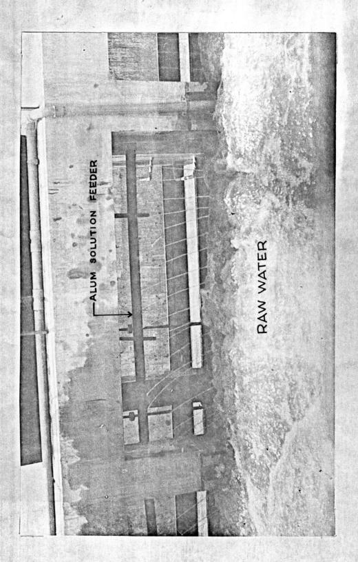
Fig. 3.2 Mixing Alum with Raw Water.
