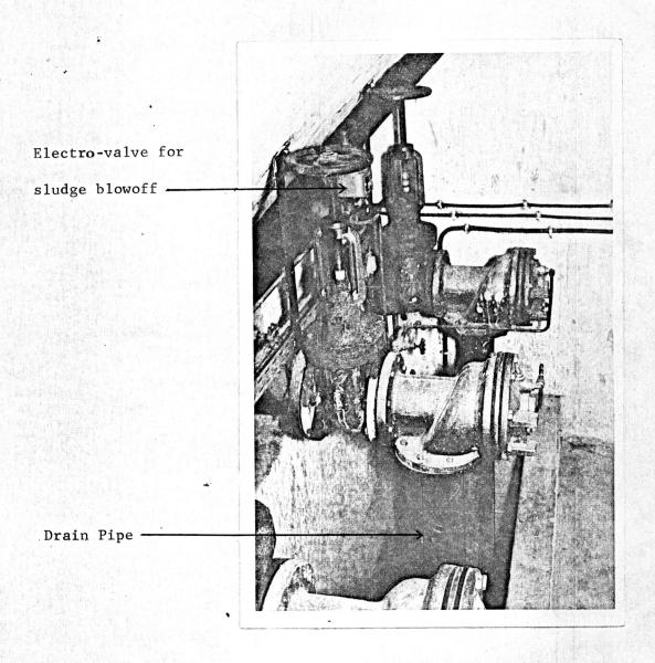
Fig. 3.4 Automatic Sludge Extraction
