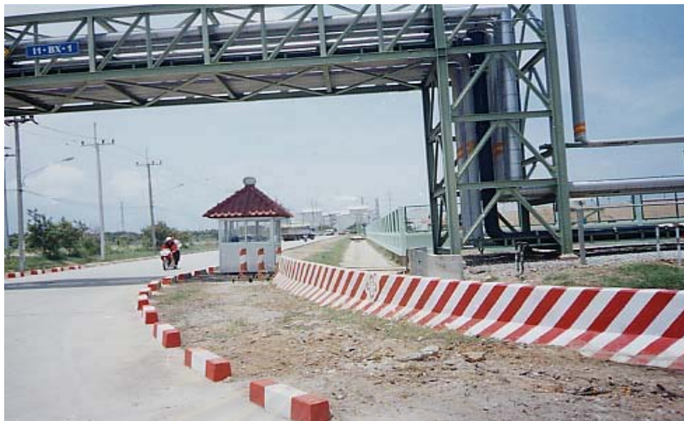
Figure 2.3: Study area with plume from petrochemical plant as a background
