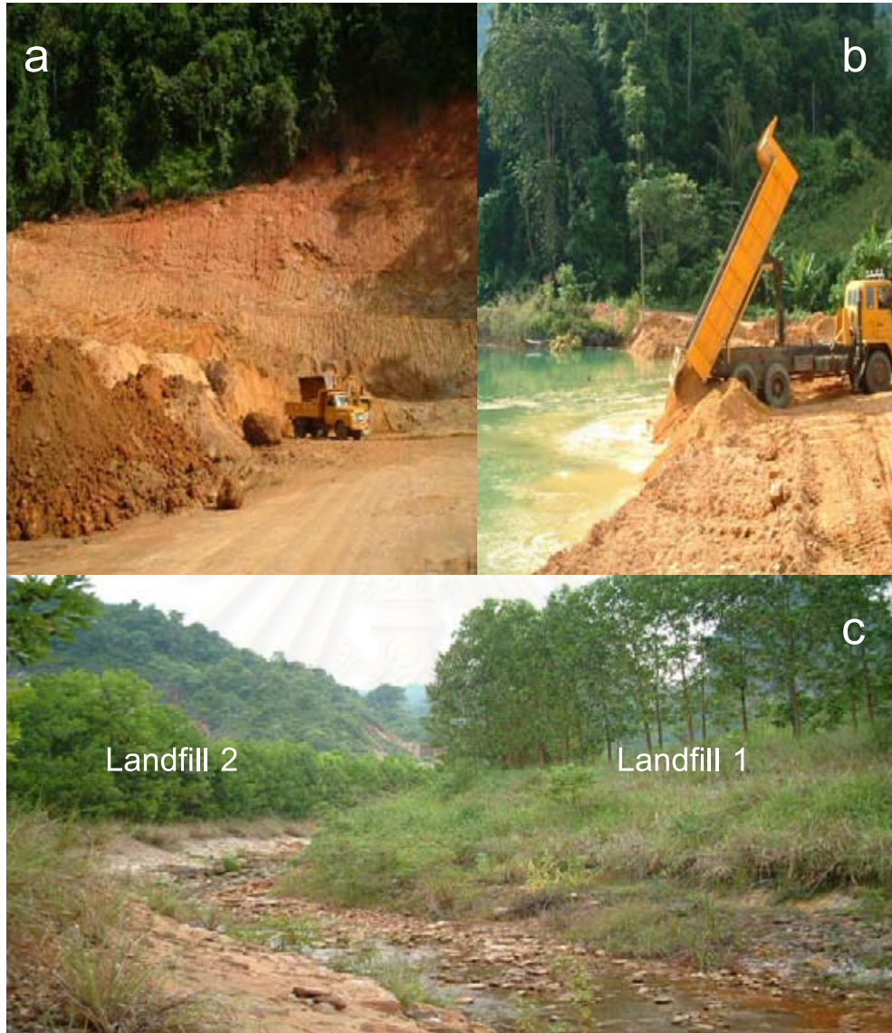
Figure 2.5 The watershed area surrounding the Euro-Thai mine was under remediation. (a) and (b) Cut- and fill- slope bench nearby the abandoned mine was taken to be dumped in the pit. (c) Landfills were built on stream banks.
