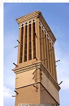
Figure 6 The wind-catcher in the hot and arid areas
