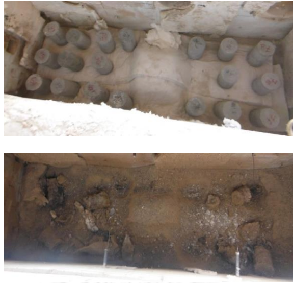
Figure 0-2 RPC cylinders (a) before fire (b) after fire
