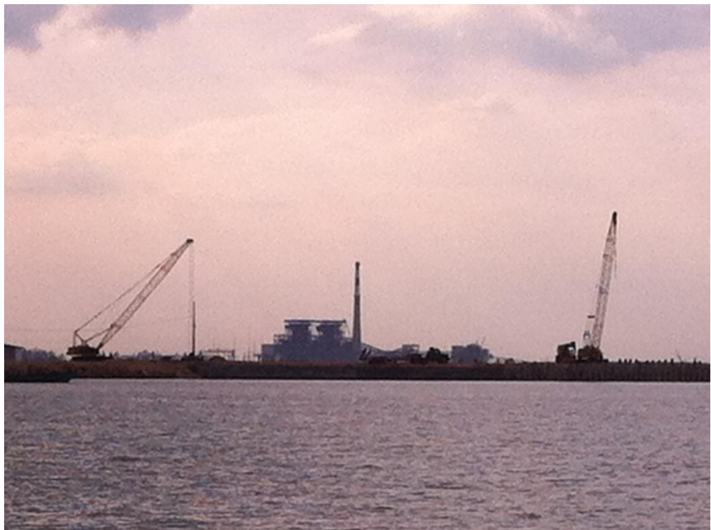
Bottom Photo: The construction of Stung Hav CFPP from Village I
