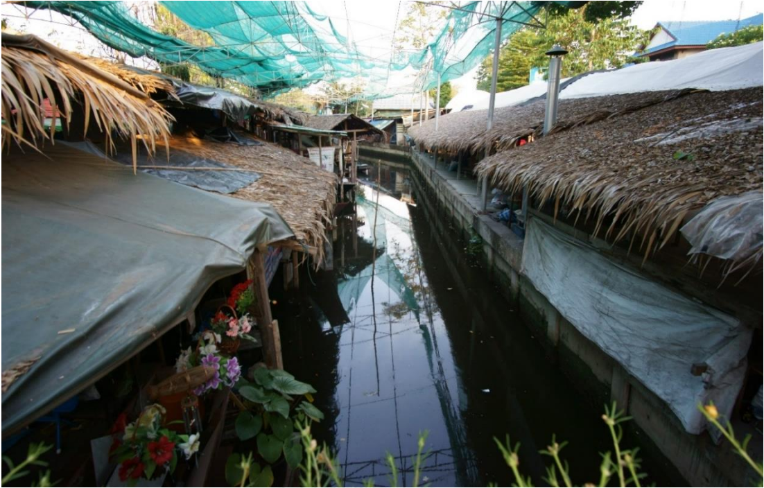
Figure 4-29 Wastewater problem in Bang Nam Pueng floating market
