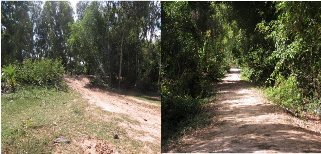
Figure 4. 2 Dike and Access Road at Doung village at Ba Baong commune in Prey Veng province.
