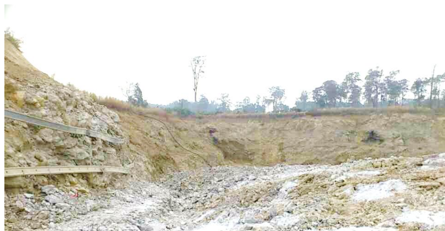
Figure 4.13 Slope face using pre-splitting method.
