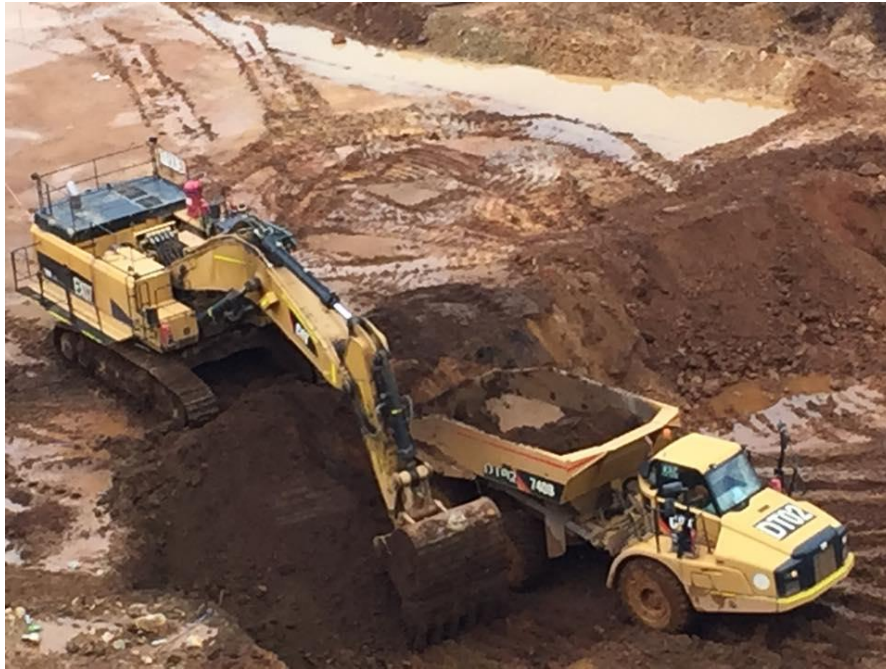
Figure 3.11 Loading and hauling system.
