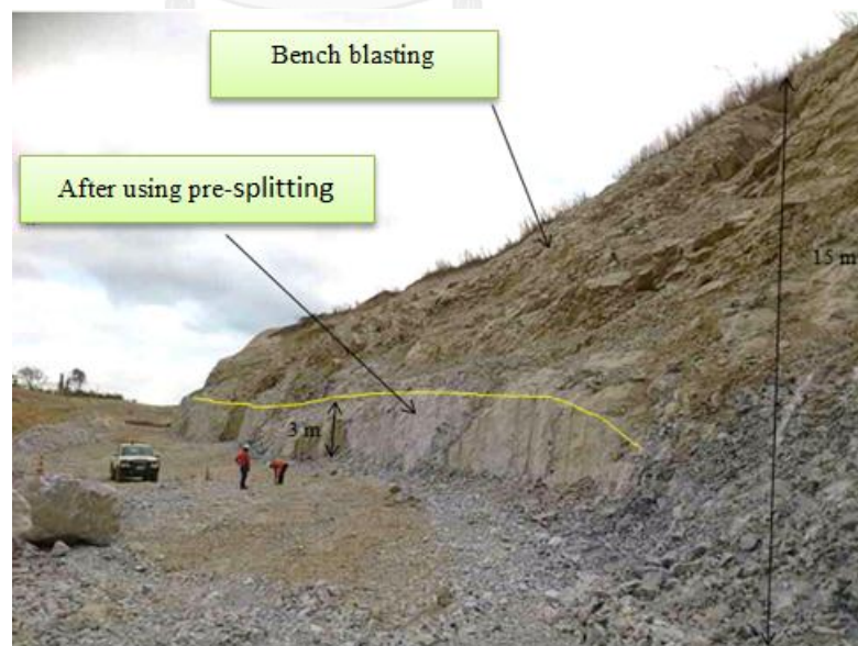
Figure 4.14 Slope face with pre-splitting method.
