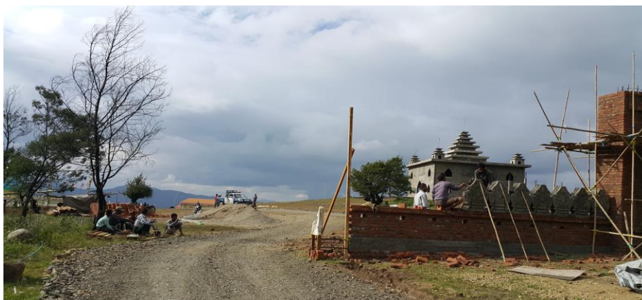
Figure 4 Pagoda Construction in the upland areas of Rung Mountain
