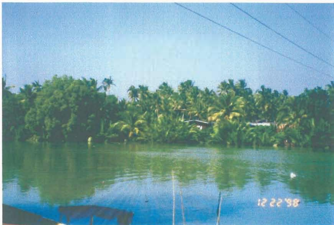
Figure 2.14 Khlong Tha Nang Sang of totally 7,500 metres long to serve as the drainage of the surface runoff from Khlong Tha Taphao.
