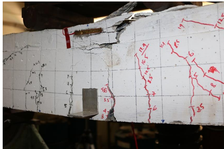
Figure 4.12 Concrete crushing failure
