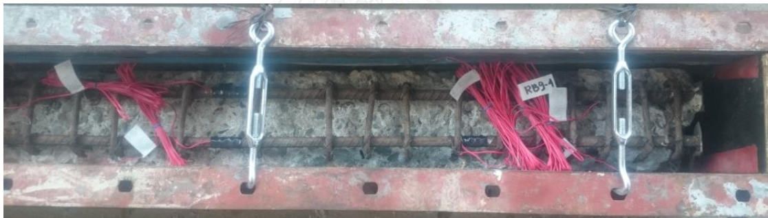
(a) Repairing set-up
