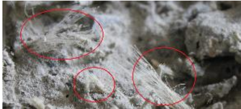
(a) Rupture failure of 40S specimen
