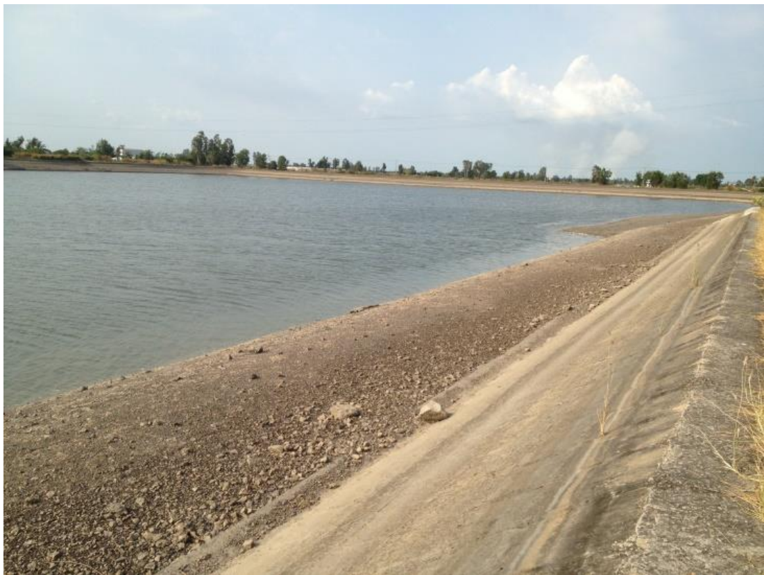
Figure 16: The 500,000\text{m}^3 pond was out of water in April 2016
