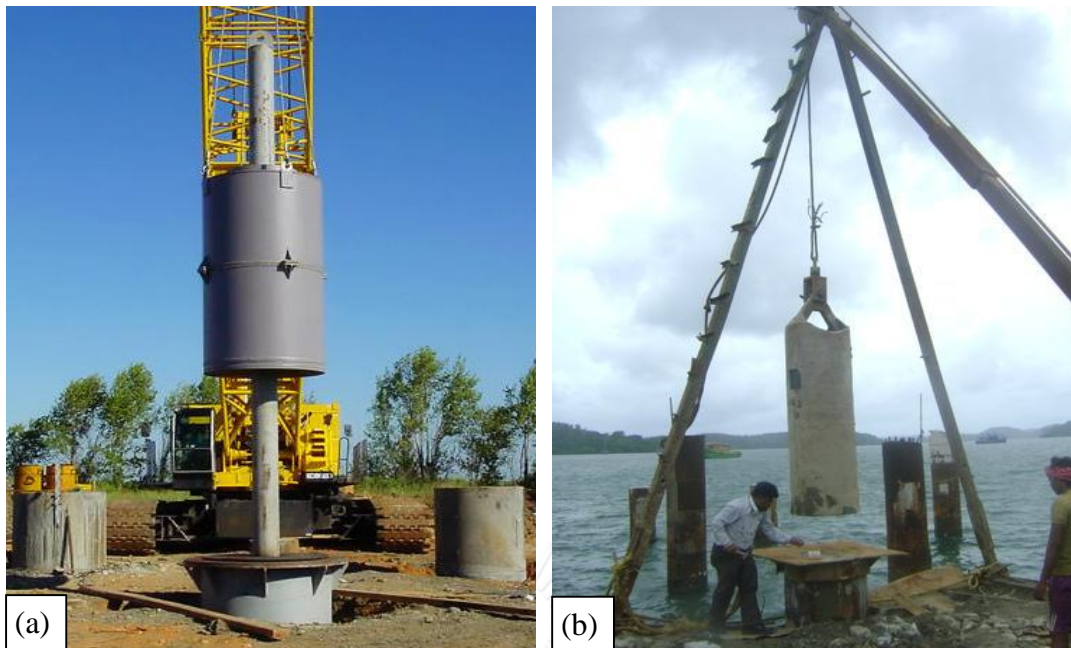
Figure 2.3 Dynamic pile load tests by a drop weight, (a) with a guiding system 1 , (b) without a guiding system 2 .
