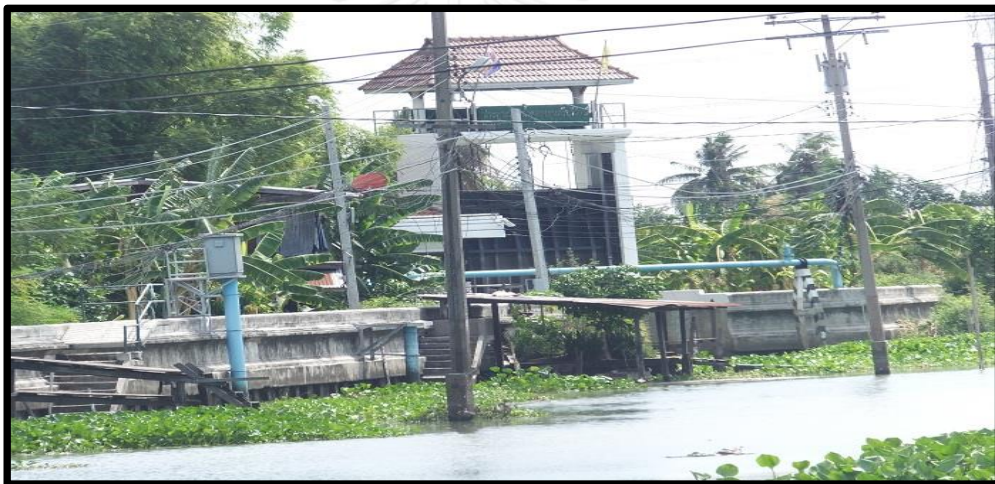
Figure 6: Khunsriborirak Sluiceway ( 12 August 2015 )
