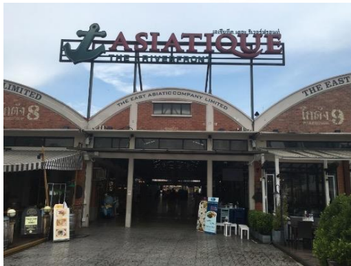
Figure 3. Middle arch Maintaining the Original Style
