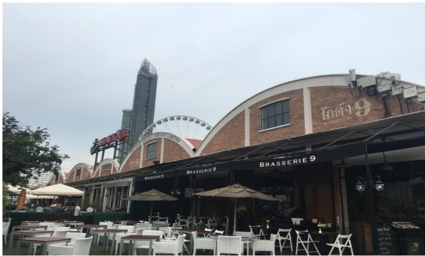
Figure 2. Five Concrete Framed Arched Brick Structures Renovated as Bars and Restaurants
