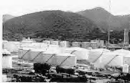
Figure 1 Process plant and storage plant in the refinery
