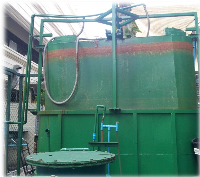
Figure 3.6 Gas holding tank (floating drum)
