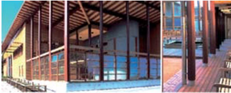
Figure 2. 12 (Left) Two-story wood building with simple roof forms but sufficient detailing of fence, shading devices and long eaves to provide visual richness; (Right) Large canopies between the inside and outside increases the spatial experience and allow children to play safely on all sides of the building. (Hosmarinpuisto School and Day Care Center, Espoo, Finland)
