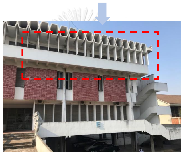
Figure 2. 48 . Interior space with opening windows to allow aeration, with double walls serving as a shield against direct sunlight
