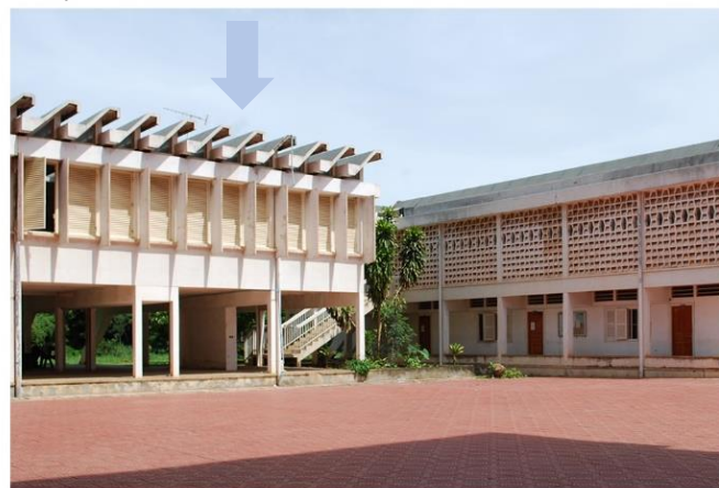
Figure 2. 50 Diagram analysis showing the skylight design to gain indirect sunlight and allow cross ventilation in the classroom
