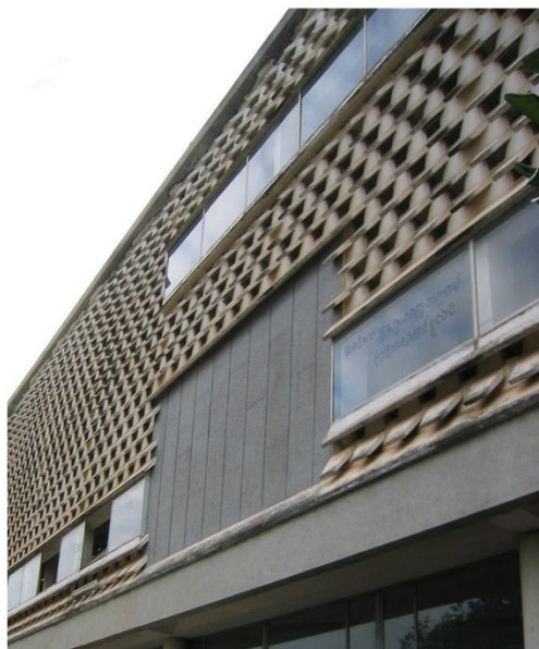
1960s ventilation block
