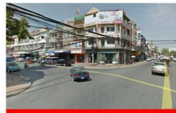
Figure 12. View from west elevation (Source: Google Earth)
