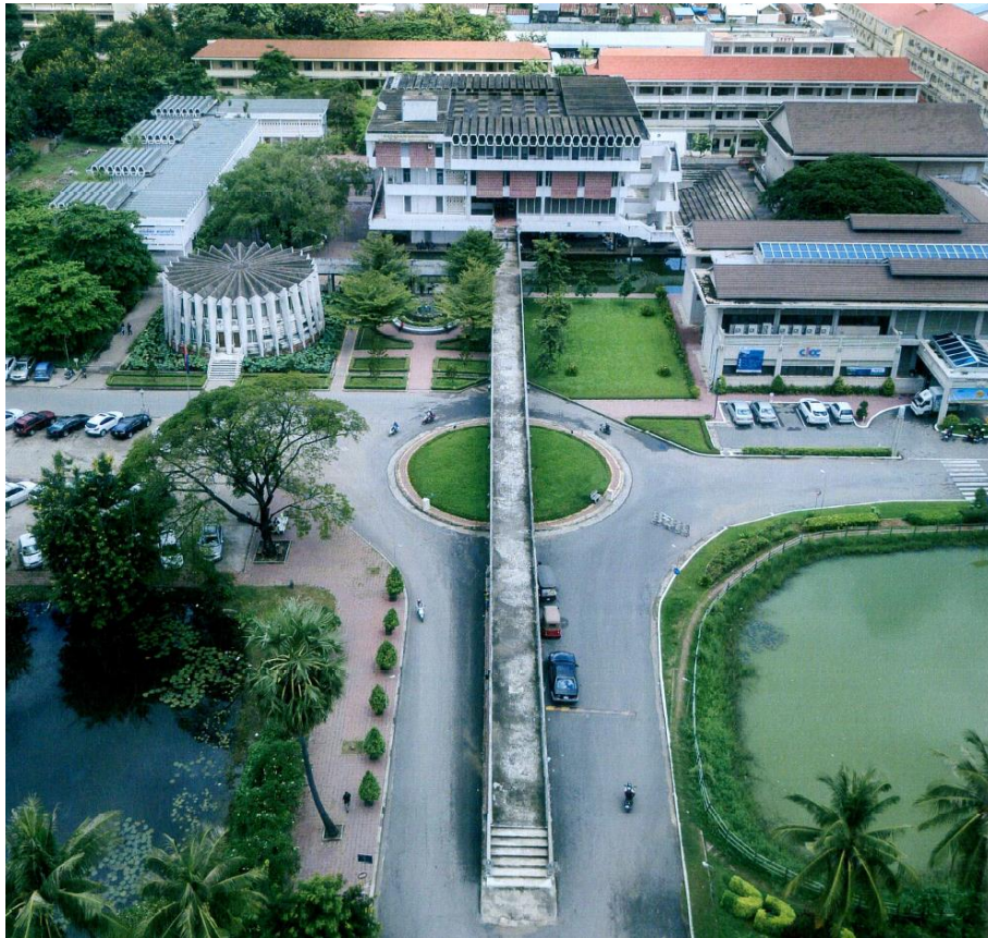
Figure 2. 38 The library and classroom at the west of the principal hall, with naga statues beautifying the handrails and elevated side walk connecting it to the classroom (source: A+U Magazine)
