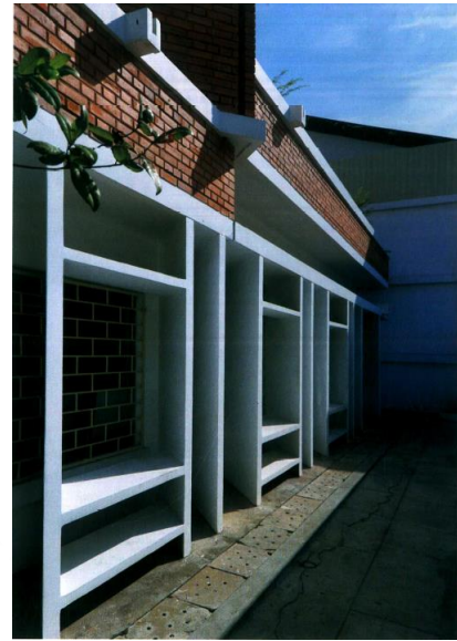
Figure 2. 75 Concrete louvers on the first floor that block direct sunlight (A+U Magazine)
