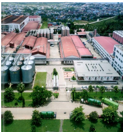
Bird eye view from the east: Masterplan of the factory site (source: A+U Magazine)
