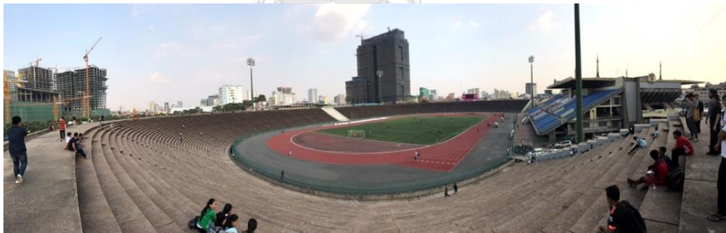
Figure 2. 26 Eastern slope of the outdoor arena (taken by author, 08 March 2018)
