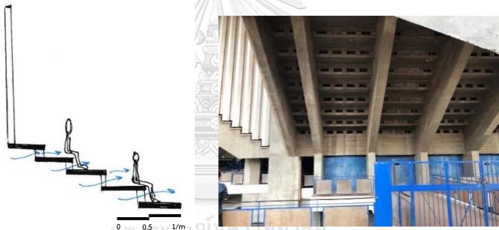
Figure 2. 21 The hole punches under of the audience's seats allow soft lighting and ventilation in the indoor arena (photo taken by the author on March 8, 2018)
