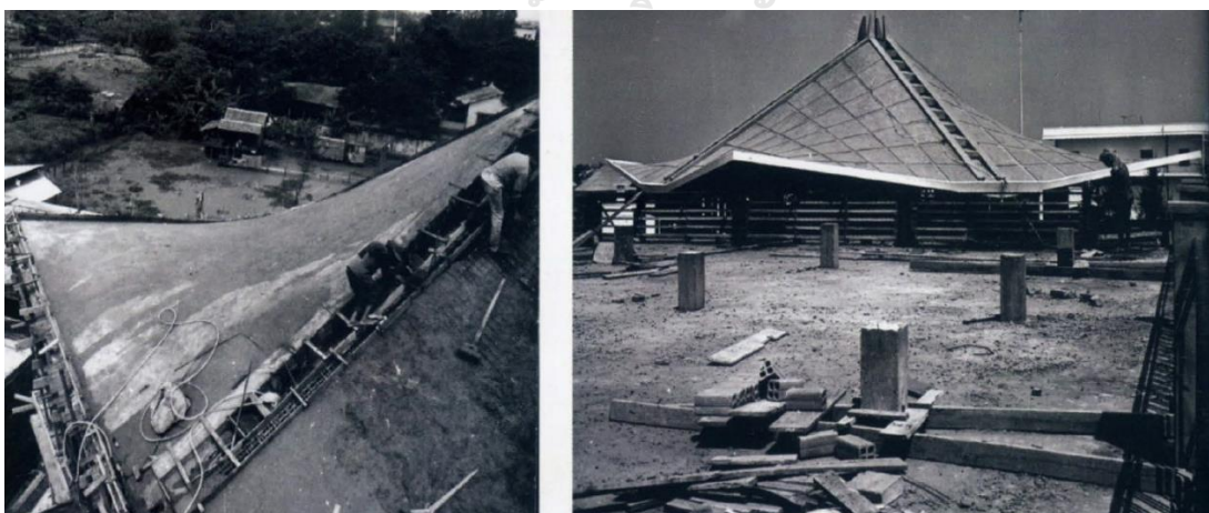
Figure 2. 74 Double roof concrete shell structure (source: New Khmer Architecture book)
