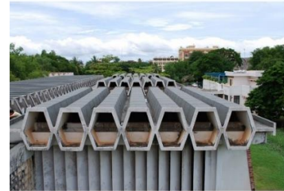
Figure 2. 49 Honeycomb double roof provides insulation against heat from sunlight by allowing it to flow through the two-layered structure
