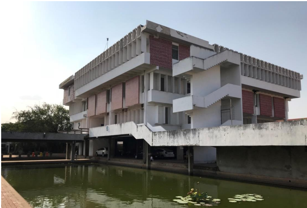
Figure 2. 37 Teacher Training College main building (taken by author, 08 March 2018)
