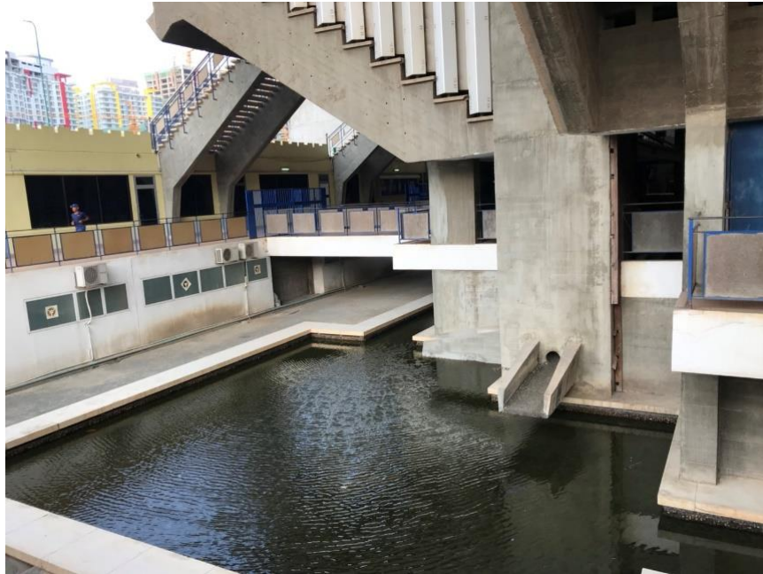
Figure 2. 25 Scupper with a vile in the middle of the column to collect rainwater from the roof (taken by author, 08 March 2018)
