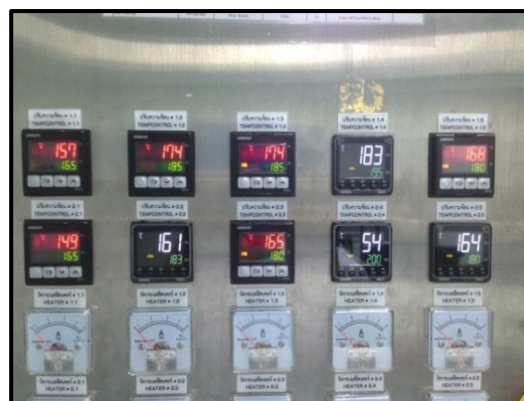
Figure 5.6: Sealing machine regulator
