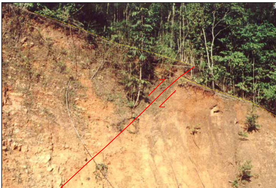
Figure 3.29 Close –up view of Ban Namtok Erawan showing an offset of surface indicating to reverse fault.
