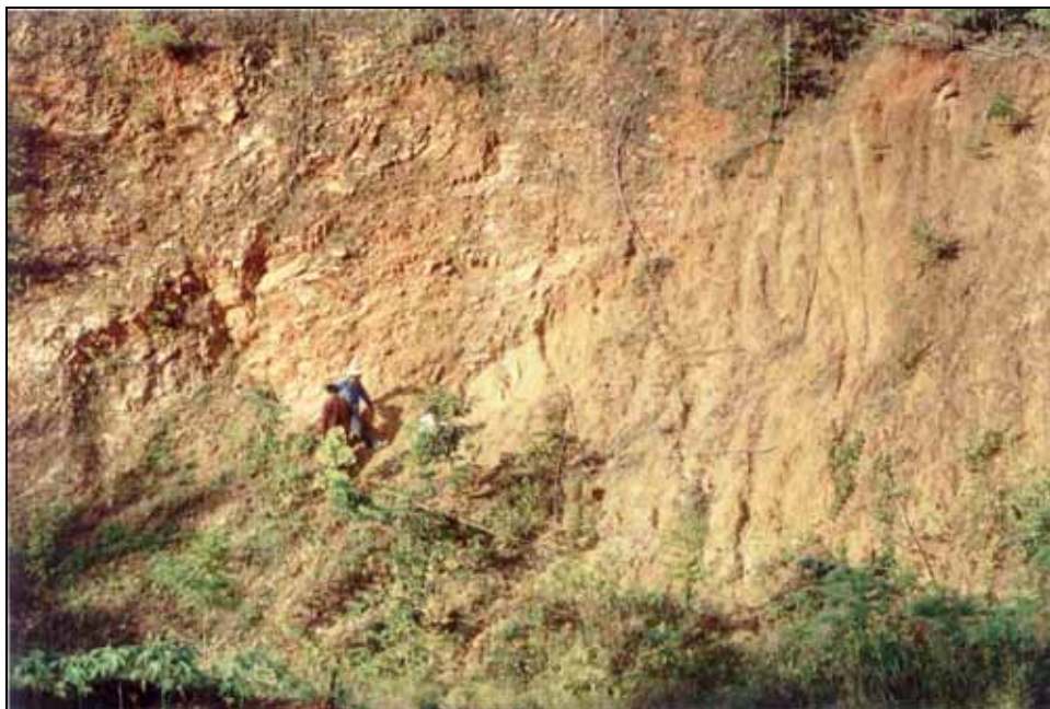
Figure 3.28 Road cut exposure showing a major fault whose plane is N60W strike and 35° dip at Ban Namtok Erawan, view looking N65°E.
