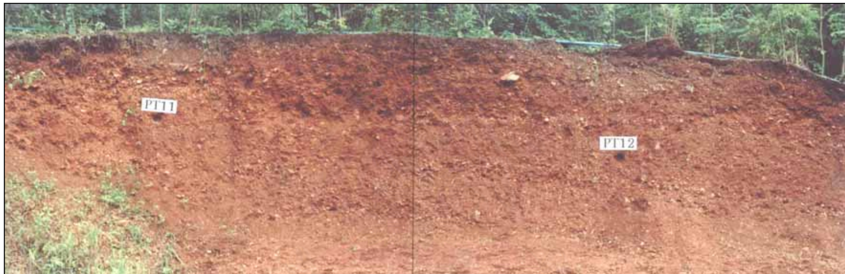
Figure 4.16 Stratigraphy of young, unconsolidated sediment deposits on the southeast trenching wall in Ban Pha Tawan II Trench , Showing location of samples for TL-dating in the fine-grained sediment layer.
