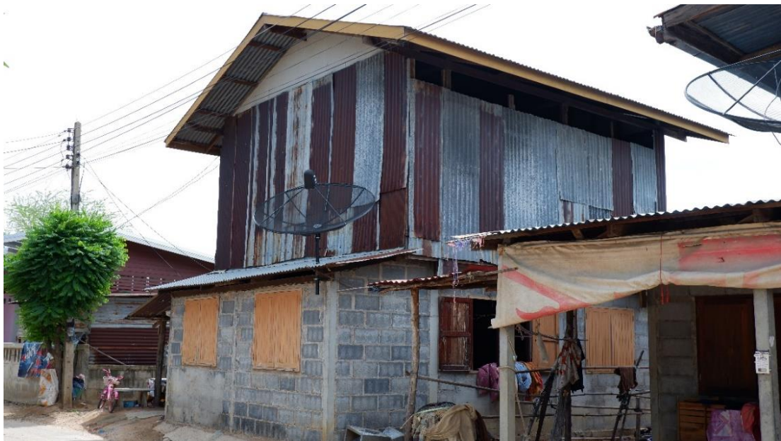
Figure 56. House no.137 in year 2019 Source: photograph by Benjarat Prompen
