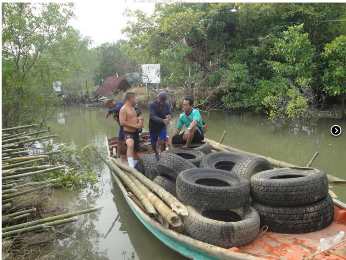
Figure 34. The villagers carry tires to build tire cubes for protecting shoreline Source: website of Ban Pred Nai
