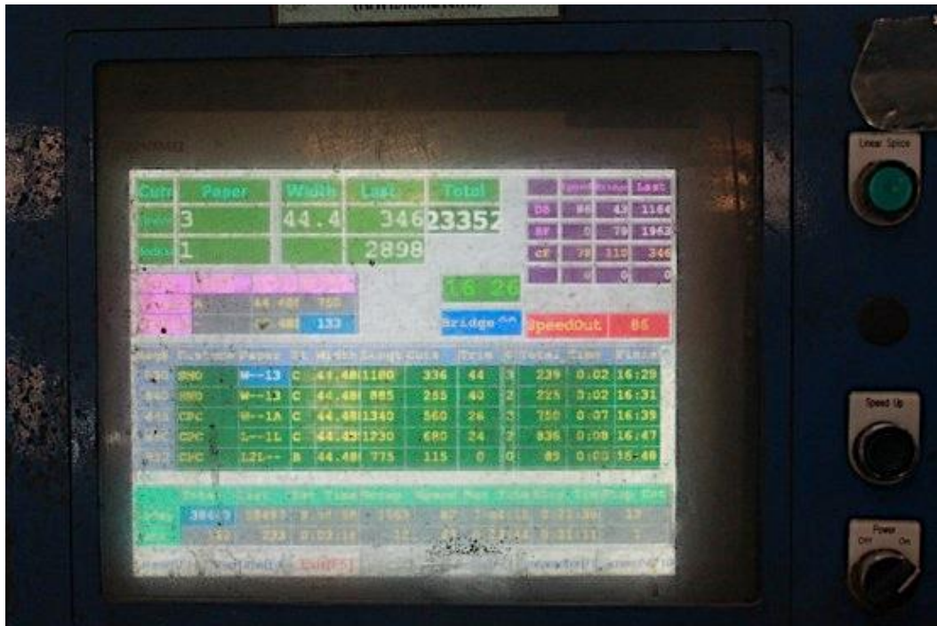
Figure 5.49: Speed Control Monitor
