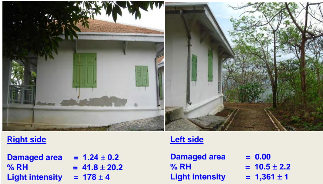
Figure 4.10 The comparative of abiotic factors affecting on the right and left sides of Apirom residence
