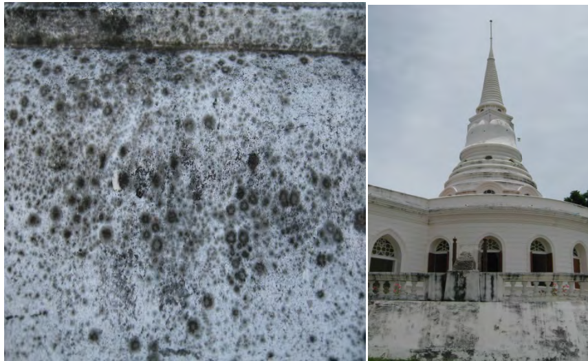
Figure 5.4 The characterization of fungi stains at Aussadangkhaniimit Temple
