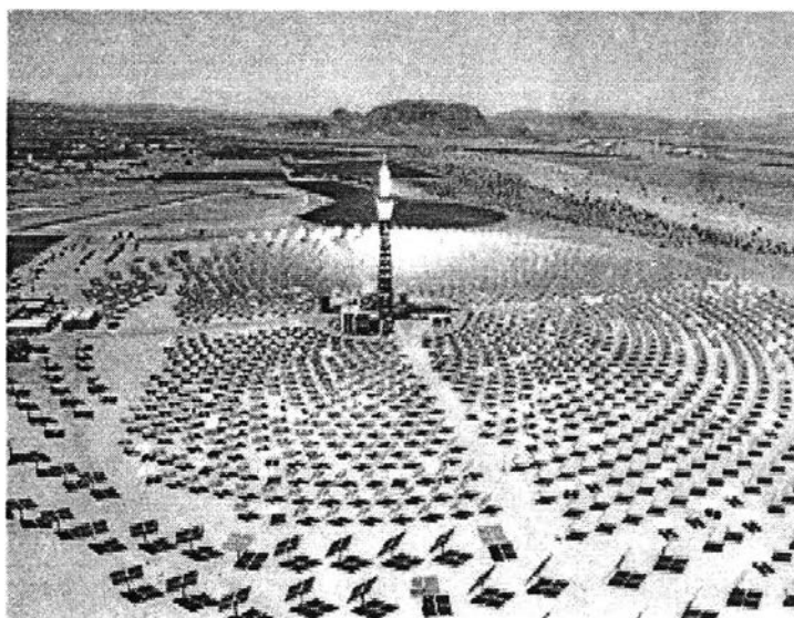
Figure 2.7: The central receiver power plant Solar One at Barstow, USA
