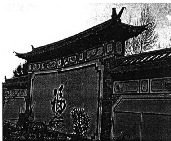
3.3, A Bai house wall
