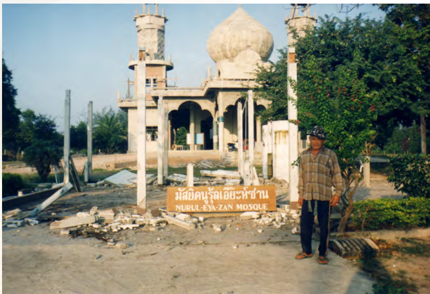
Nurul Iyasan Mosque in Cha-Am district, Petchaburi province, under construction
