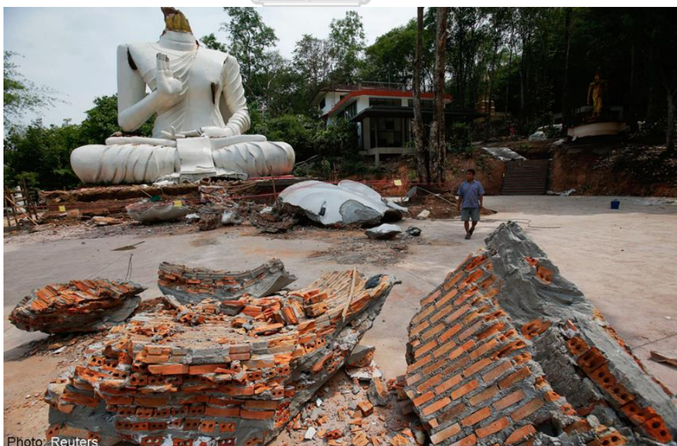
Figure 1.4. The photo shows the damage establishment by The M_w -6.3 Mae Lao earthquake on May 5 th , 2014, in Chiang Rai, Thailand ( https://www.asiaone.com/ )
