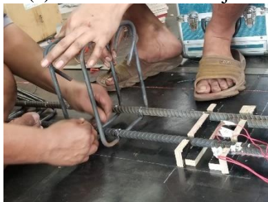
(c) Tying stirrups to bottom bars
