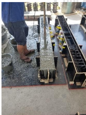
(g) Placing and compacting concrete
