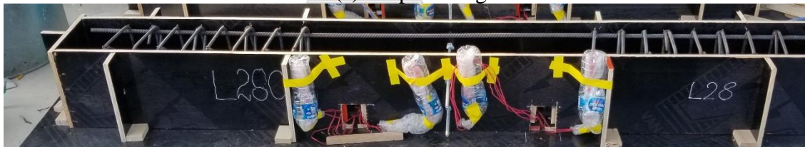
(f) Prepared cage in formwork
