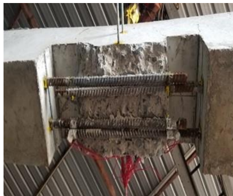
(a) Splitting failure (Type-I)
