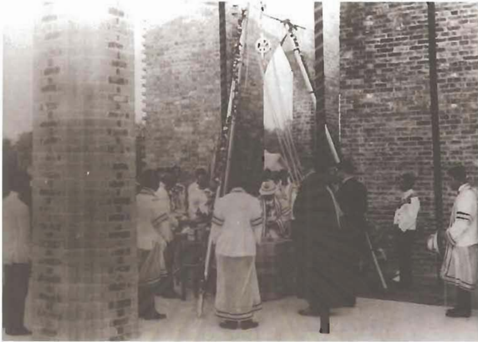
King Vajiravudh, the Royal Patron of the Civil Service College of King Chulalongkorn, laid the foundation stone of the Administration Building at 4.07 p.m. on Monday, January 3, 1916.
