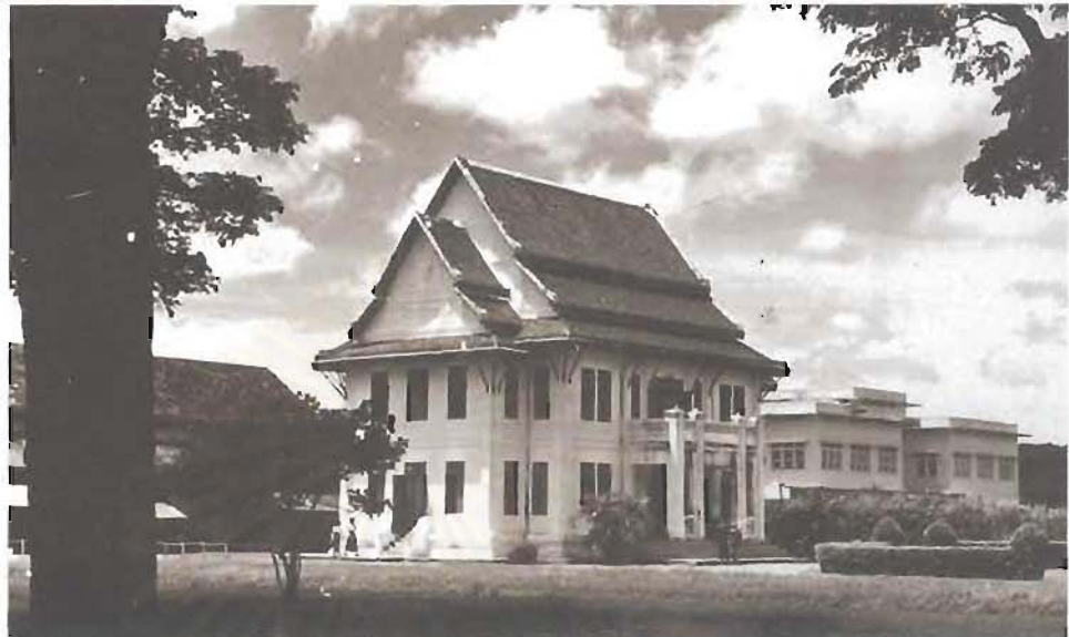
The Chakrabongse Student Union Building was completed in 1932. Prince Chula Chakrabongse provided his own fund for the construction of the building in honor of his father, Prince Chakrabongse of Bisnulok.
