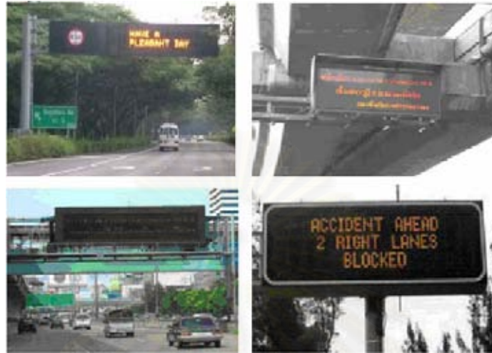
Figure 1. Variable Message Sign
