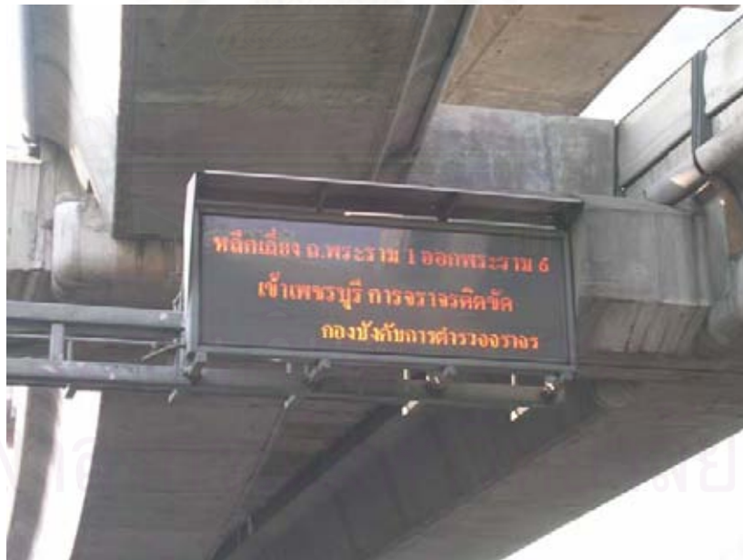
Figure 3.5 VMS located in Rama I road, Bangkok ( author )
