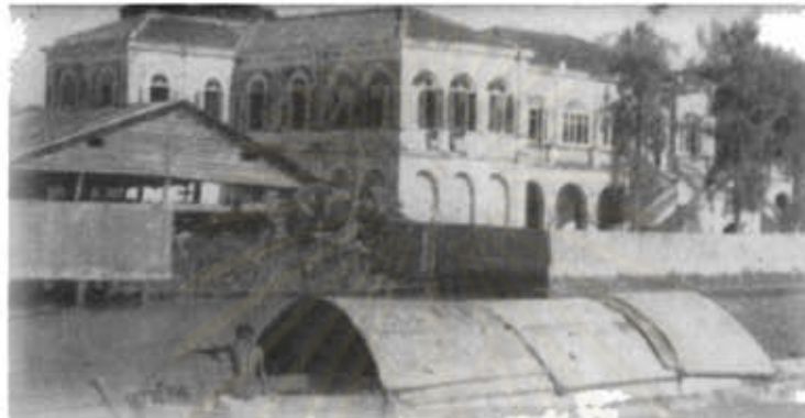
Figure 102: Ratchakarun school Bang Yee Khan, view from the Southeast
