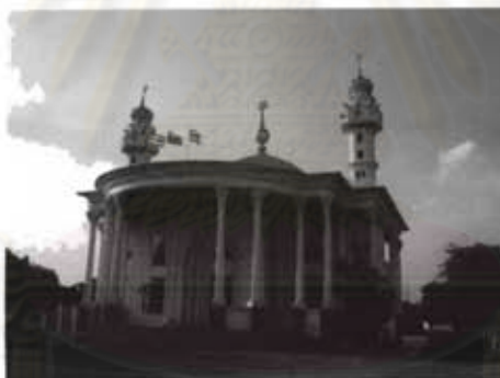
Figure 124: The Rohmatulah Mosque in front of King Rama IX Park, Srinakarin Road (Source http://www.chomthai.com/forum/view.php?qID=2161 retrieved on 24-6-2010)
