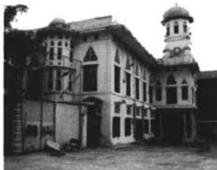
Figure 110: The Jakkapong Mosque during the renovation (Source: Adis Raksamani, 2008: 128)
