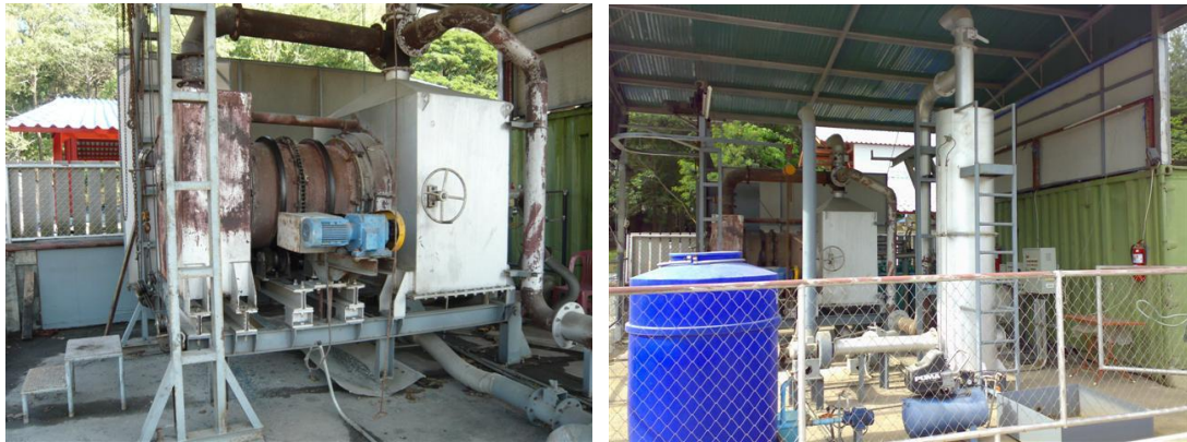
Figure 3.2: The pilot-scale rotary cement kiln
