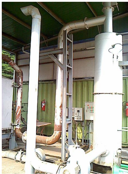
Figure A.3: The cooling tower
