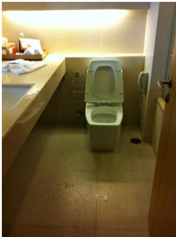
Figure IV-29: Bathroom Floor after Wiping
