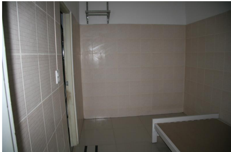
Figure III-100: Part of Area Prepared for Spa Service
