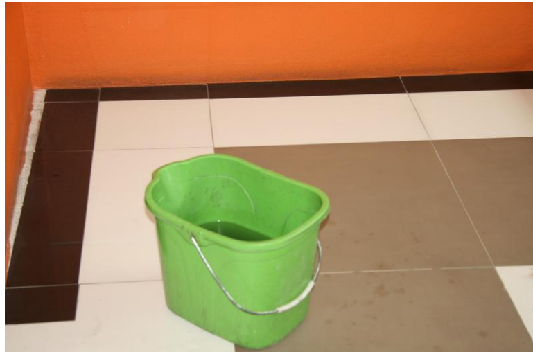
Figure III-86: Water Bucket and Splashed Water in the Area
