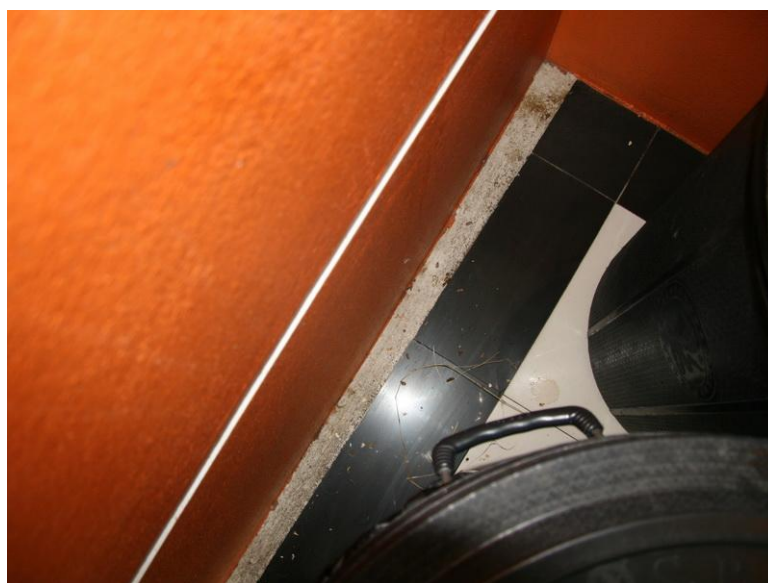
Figure III-84: Garbage Bin Area
