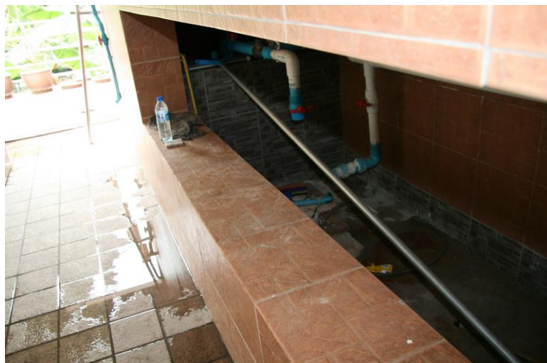
Figure III-96: Backside of Swimming Pool
