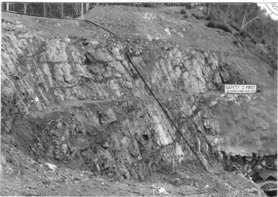
Figure 8.9 Panorama of downstream diversion tunnel.
