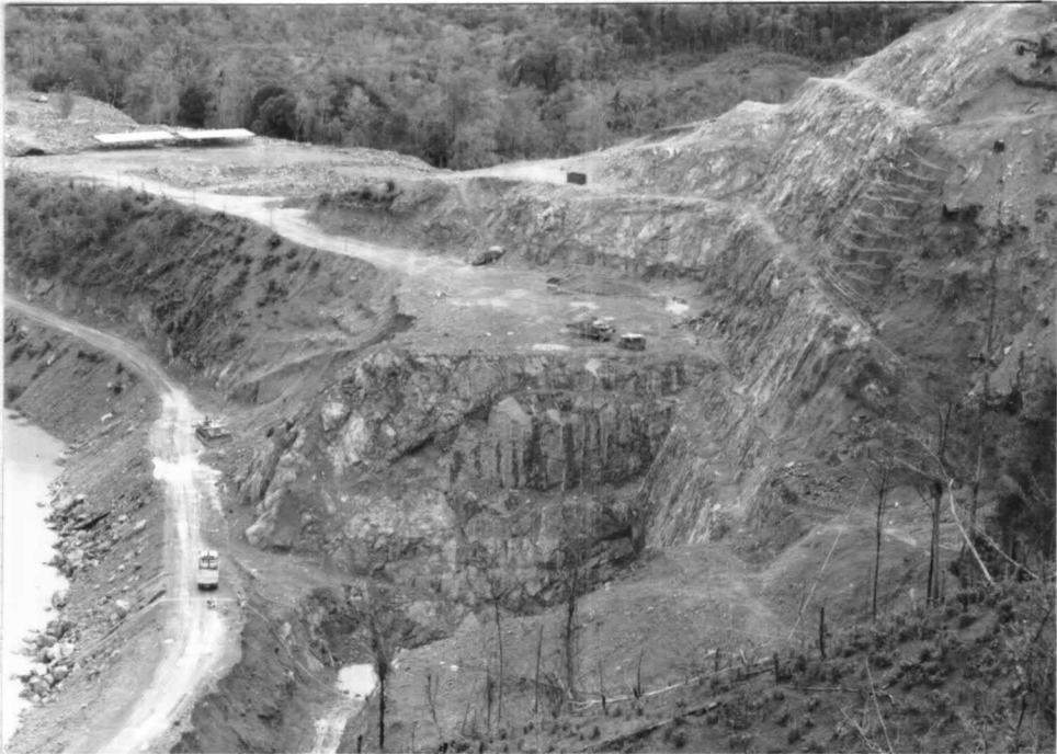
Figure 8.8 Panorama of upstream diversion tunnel.
