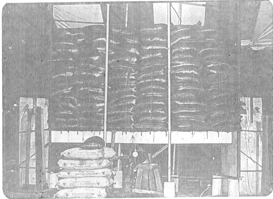
Photograph 7.9 S-beam Model at an Early Stage of Loading.
