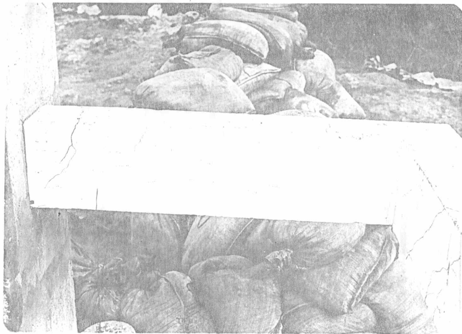
Photograph 7.19 Z-beam Model; Another View of Crack Modes.
