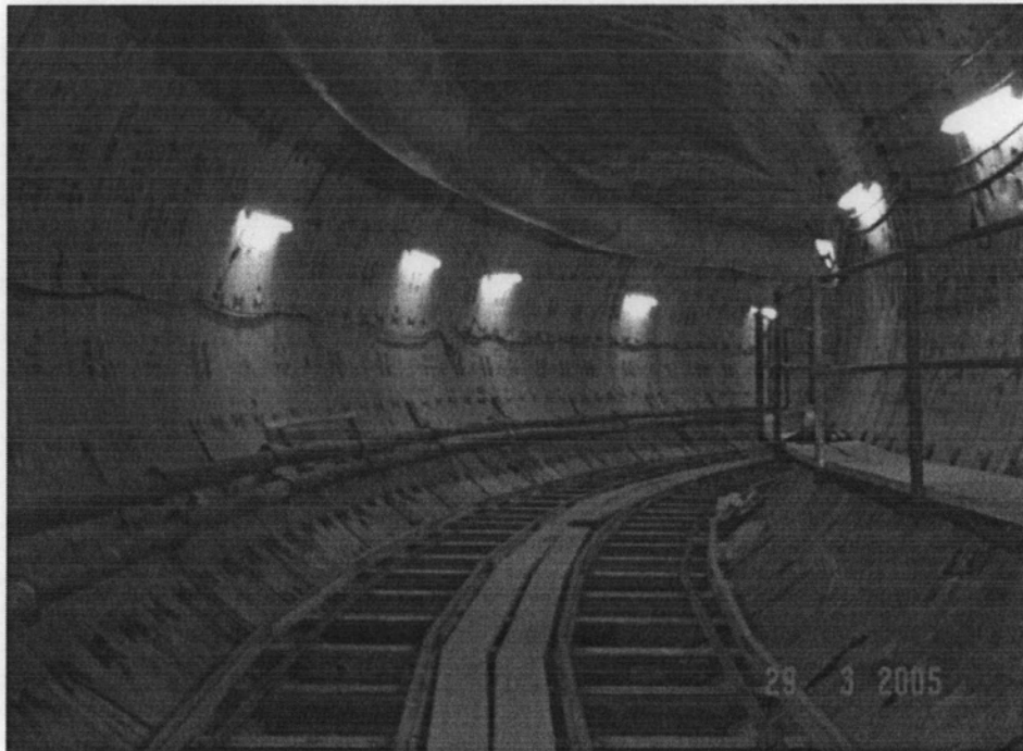
Figure 2.13 Tunnel lining after erection (BMA flood diversion project, Saensaep-Latphrao Phrakhanong)
