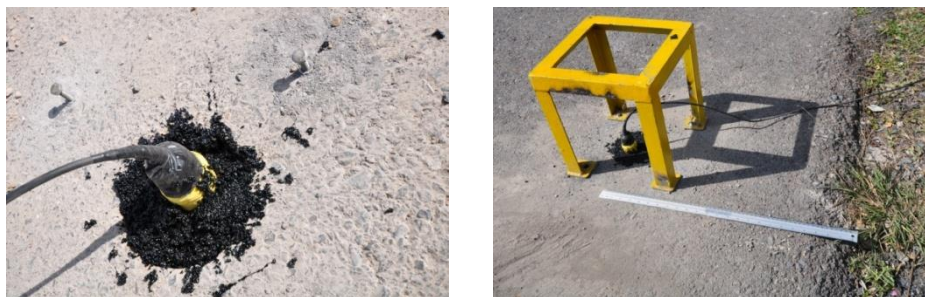
Figure 3.23 Finishing the Installation and Restoration
