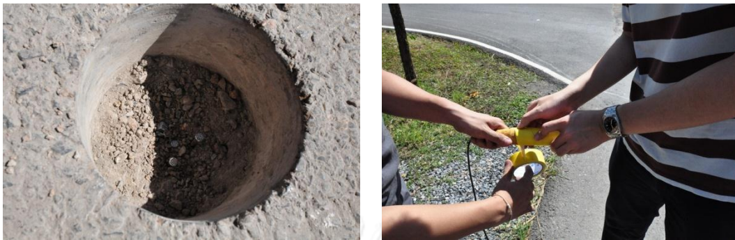
Figure 3.19 Hole and Sensor Preparation
