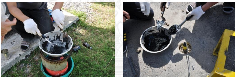
Figure 3.22 On-Site Asphalt Concrete Mixing
