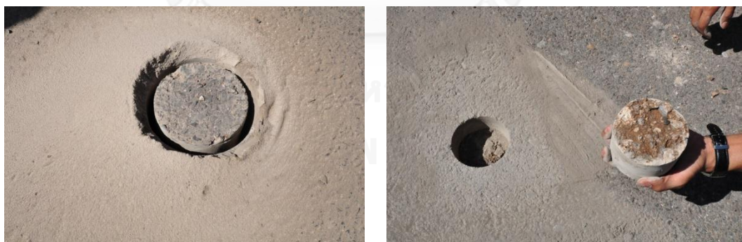
Figure 3.18 Core-Drilling Result and Spot Removal
