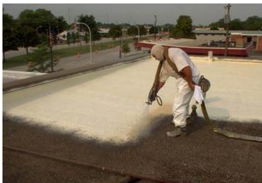
Figure a - 2 Roof-top insulation: Polyurethane foam is sprayed onto the rooftop.
